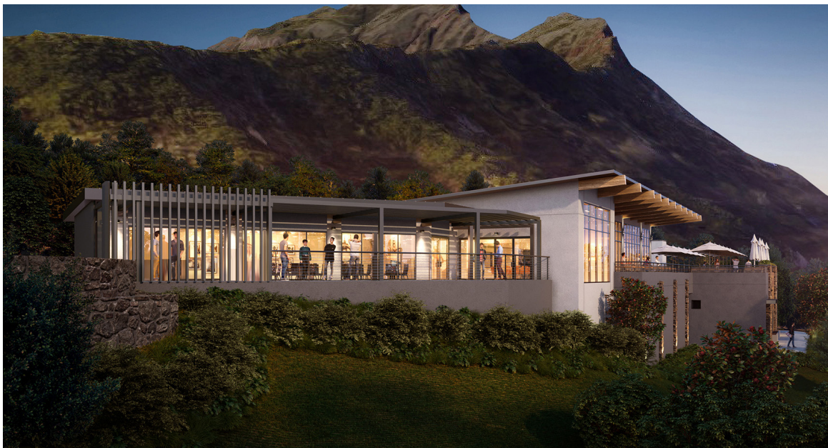
Rendering of the Kapi'olani CC Culinary Institute of the Pacific Restaurant Phase 2. Image courtesy of Ushijima Architects.
