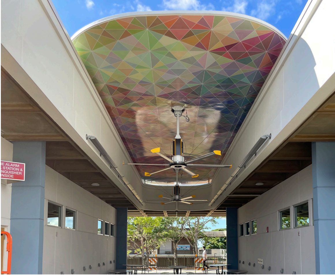
Leeward CC breezeway renovation.
