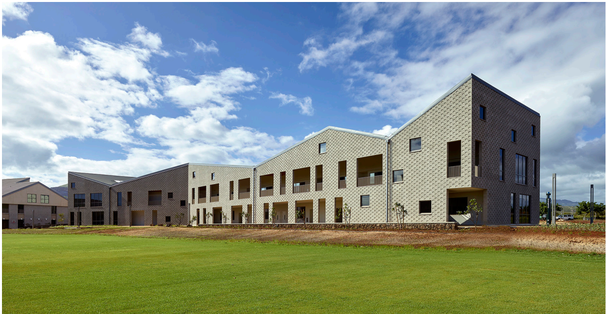
Administration and Allied Health building
