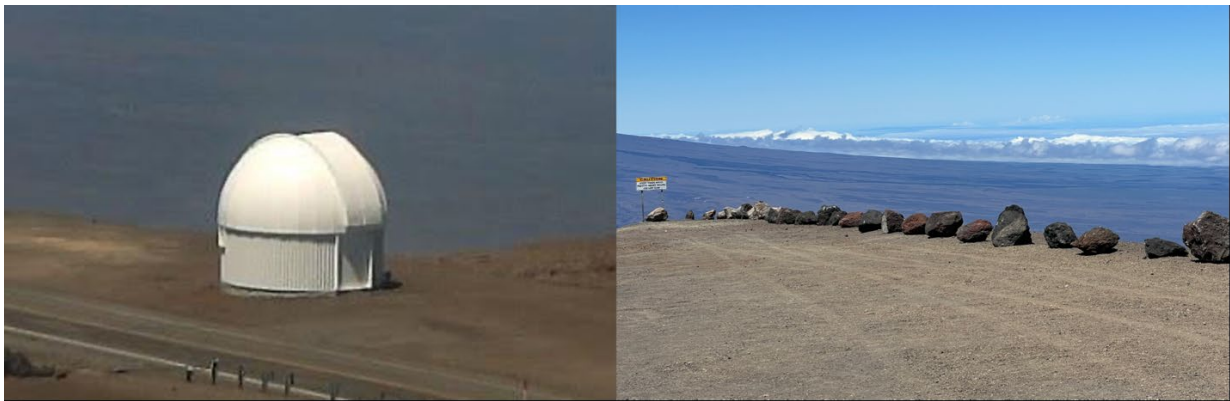
Figure 3. Hōkū Ke‘a Decommissioning: Before and After
