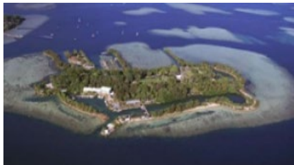
Figure 1. DC microgrid project site, Coconut Island.
