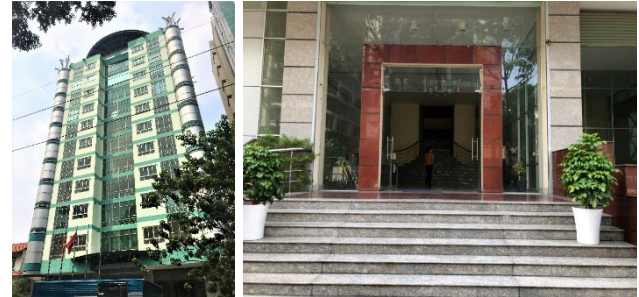
Figure 1. HCM-USTA Building, Ho Chi Minh City.
