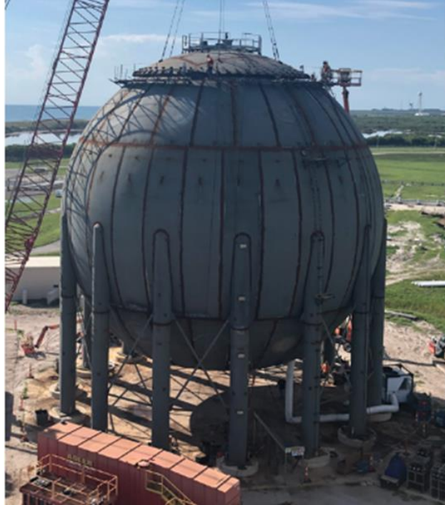
Figure 7.4. NASA 330 metric ton large-scale liquid hydrogen storage tank 16 .
