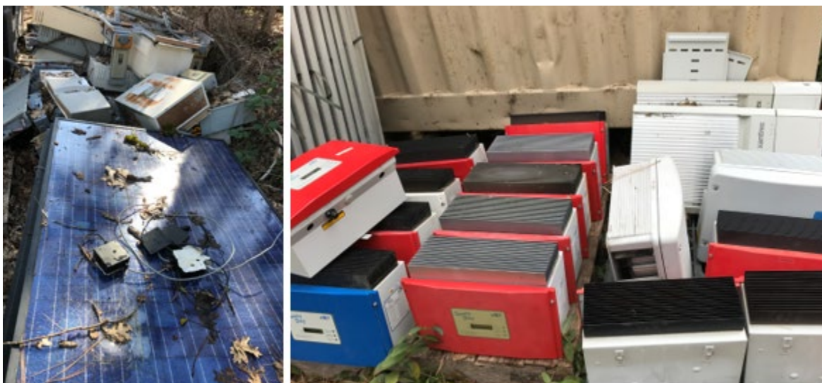
Figure 50. Images of dumped PV panels and inverters.
