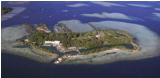
Figure 1. DC microgrid project site, Coconut Island.
