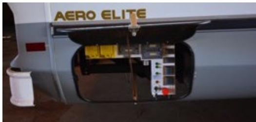
Figure 9. Bus Export Power Unit.
