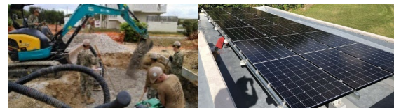
Figure 4. Project construction and new PV system.
