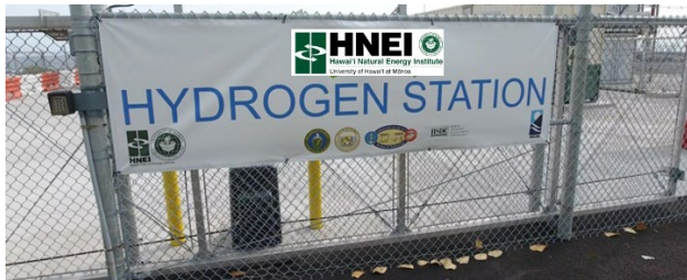
Figure 1. HNEI's NELHA Hydrogen Station.
