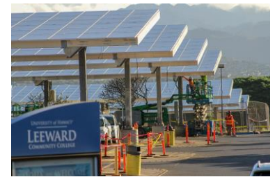
Leeward – Parking Canopy
