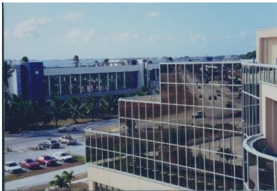
The Marshall Islands Capitol building reflects life in an urban center.
