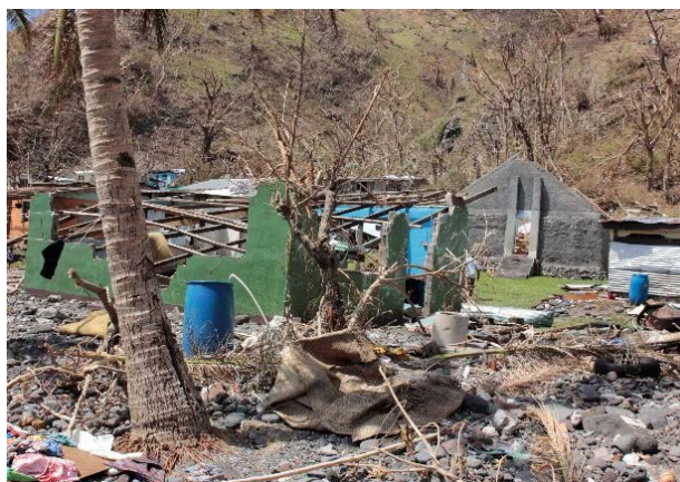
Figure 17: Example of the damage caused by Tropical Cyclone Winston.
