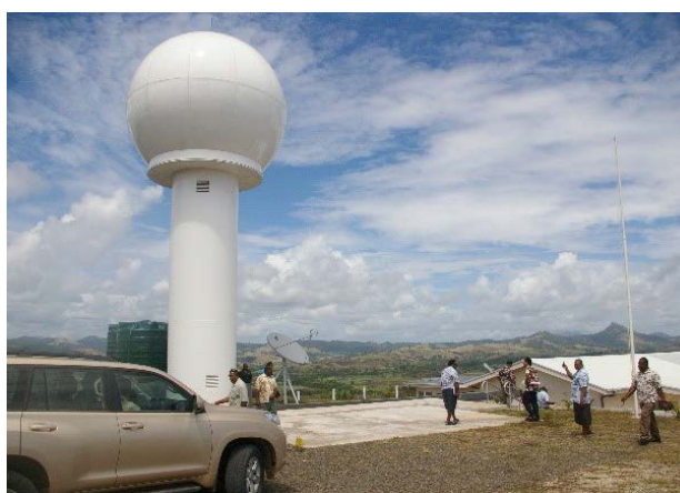
Figure 22: Vatudamu Weather station.
